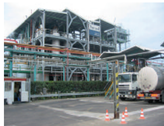
Impianto biodiesel in Malesia
