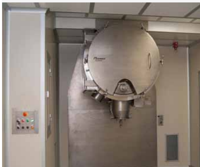
Planex System installazione presso Euticals (Lodi - MI)
