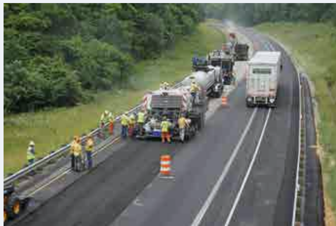
Fig. 9 The recycling process of the road pavement
