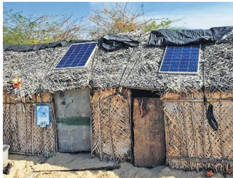
PV panels on the roof of small houses in third world countries
